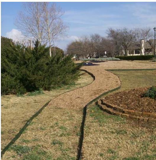
The xeriscape project in progress – 2/25/2000
