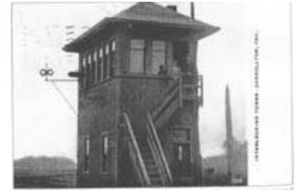
INTERLOCKING TOWER PROGRAM, PRT. An interlocking tower or switching tower was constructed near the depot. The lower portion housed the control apparatus for the rail head signals and switches. The upper story of the tower provided better visibility of the tracks and incoming and outgoing trains for the operator. © Courtesy of Ed Williams?
